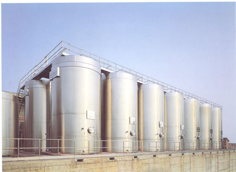
■ Storage special tanks.
